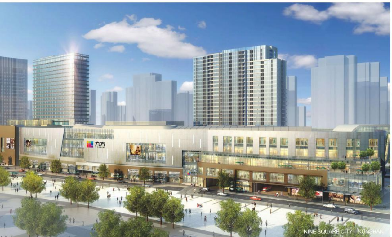
AVIC CENTRAL SQUARE—LUOYANG
